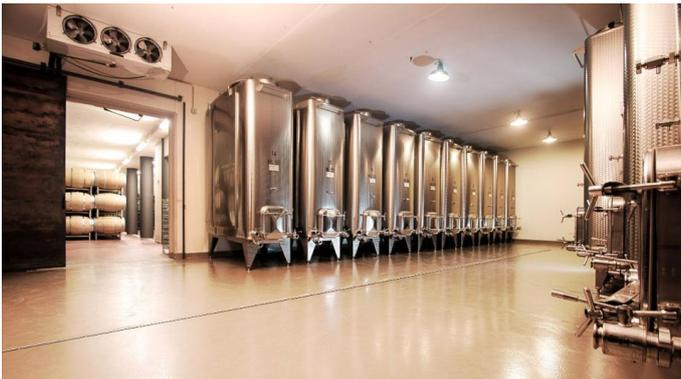
Temperature-controlled stainless steel tanks are used to preserve the freshness of newly pressed ...
